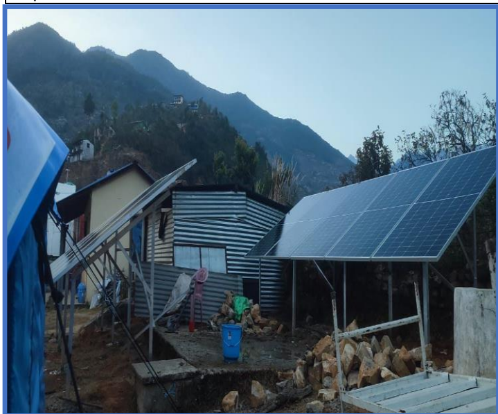
Installation of 5.45 KW solar panel at Barekot & Junichande Birthing Centres
